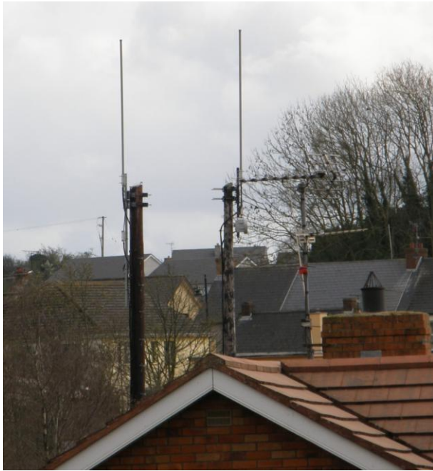
Transmitter Site Photo
